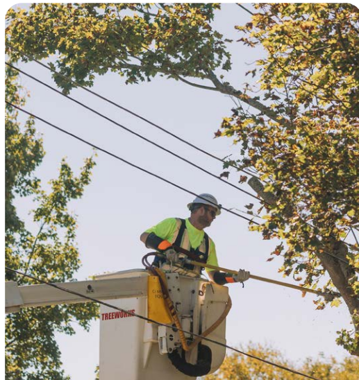
Trees are trimmed back from Nova Scotia Power lines. Proactive vegetation management is critical as storms become increasingly severe and more frequent.
